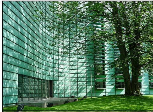
Copper façade of Nordic Embassy, Berlin
